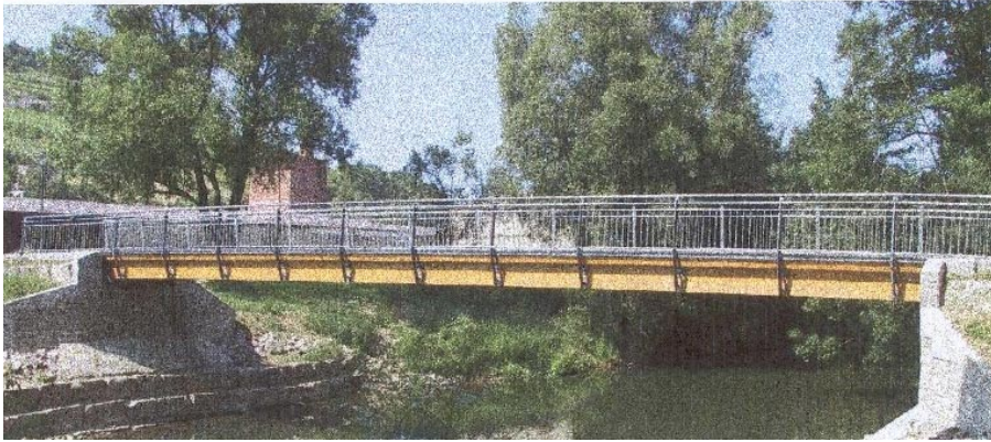
Fig. 8 Pedestrian and cyclist bridge "Heiliges Wöhr" at Weikersheim
