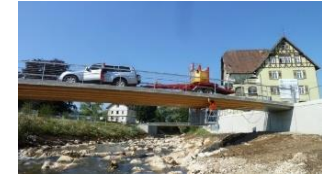
TCC with notches; integral abutments
