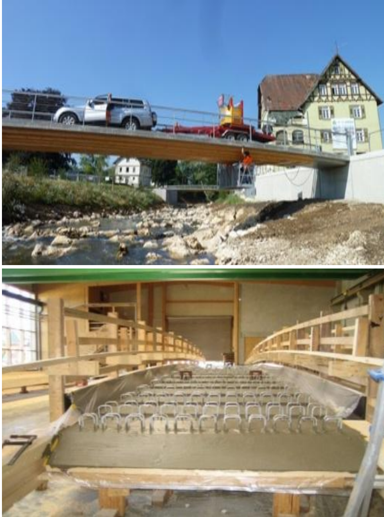
Figure 7. Examples of integral timber bridge designs, Source: Matthias Gerold
