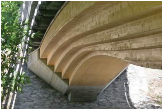
Figure 7. Example of an integral timber bridge without bearings and transition joints (photo: Schaffitzel Holzindustrie)
